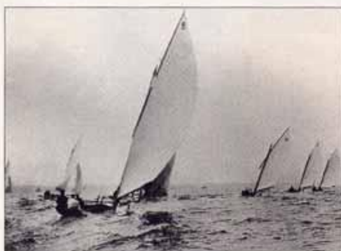
Previous page: Moyana , a 52-foot Linear Rater built in 1906, had the vast sail-area and overhanging boom typical of the class.
